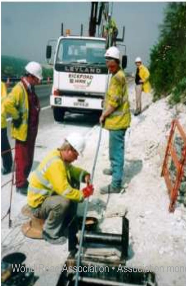
Pulling a cable
