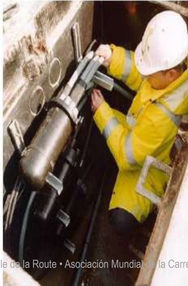
A Below Ground Joint
